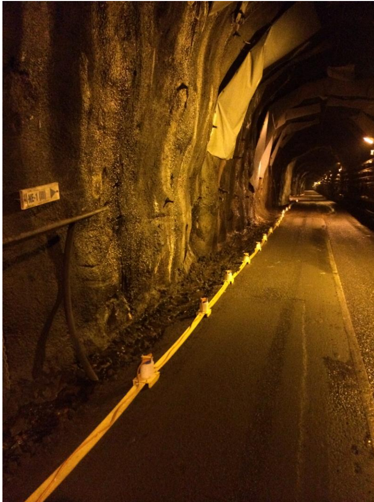
Figure 10. Photo showing the deployment of the landstreamer in the Äspö tunnel intersecting the NE1 fracture system. The experiment was done using a tunnel-surface-tunnel seismic experiment.
